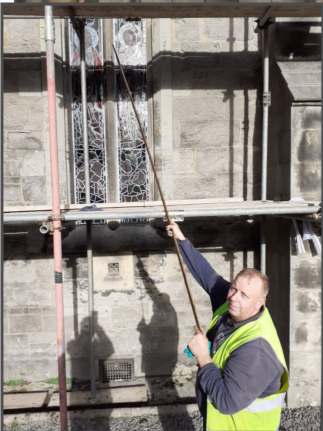
Dermot Ferris pointing out the loose mullion.
