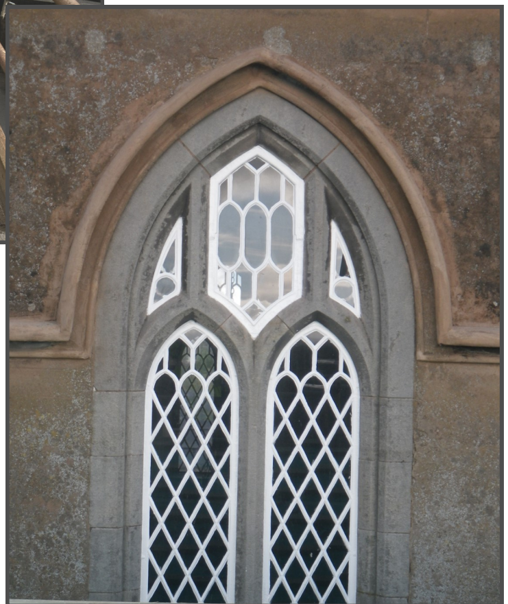
A restored and freshly painted high level window. Plaster work on the high level windows required repair, due to age and weather damage.
